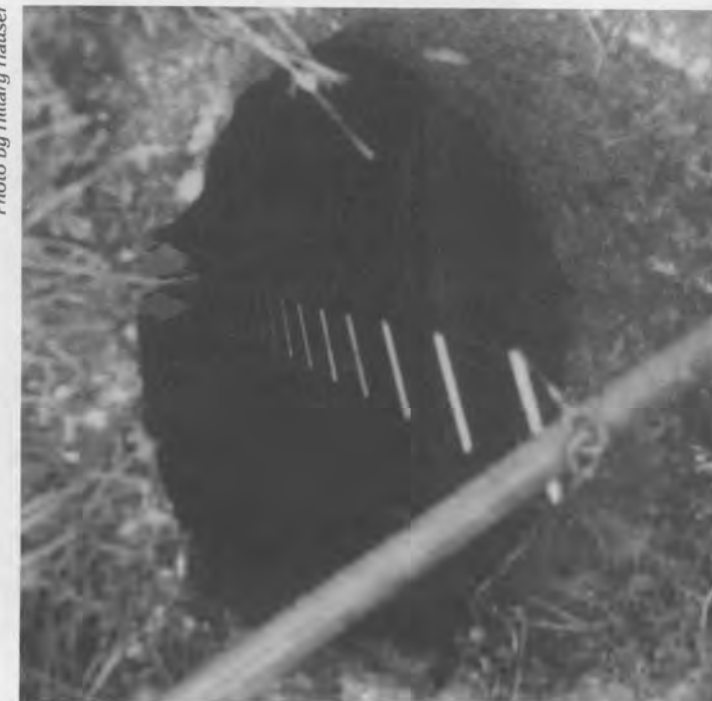
A topside view of the ladder leading down into the Shaft.
